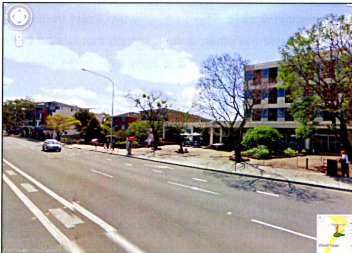
Photo 11: Hawkesbury Road looking northeast from the subject site
